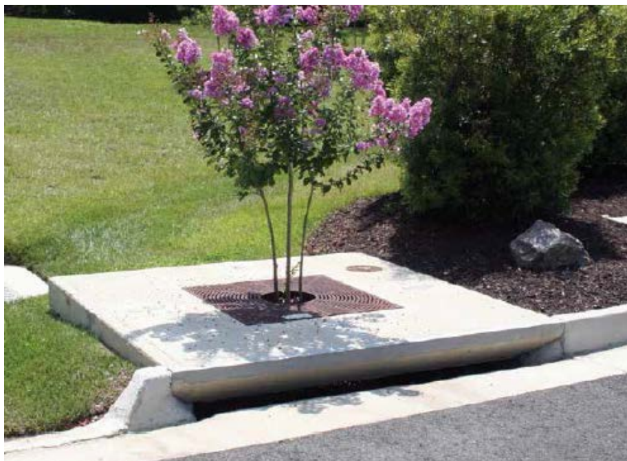
Figure 7. Example of a Biofiltration System.
