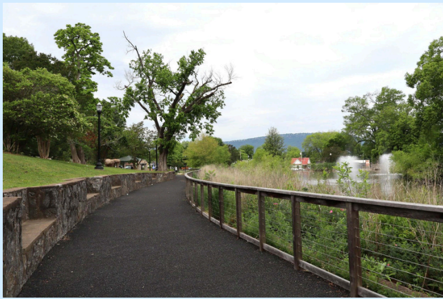
Photo 3. Pervious pavement track that circles the pond at East Lake Park.
